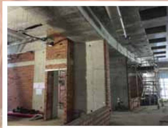
L1 Lift Lobby
